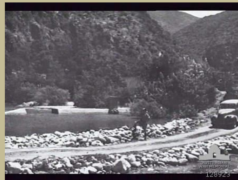
DAMOUR AREA, SYRIA. 1941-07. PART OF THE DETOUR CONSTRUCTED AROUND THE DEMOLISHED BRIDGE ACROSS THE DAMOUR RIVER ON THE BEIT ED DINE ROAD BY 2/6TH FIELD COMPANY TO TAKE ANTI-TANK GUNS
