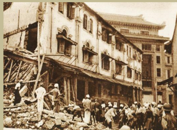
Singapore buildings damaged by Japanese Air Raids
