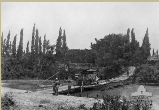
Temporary bridge across the Litani River built by the 2/6th Engineers
