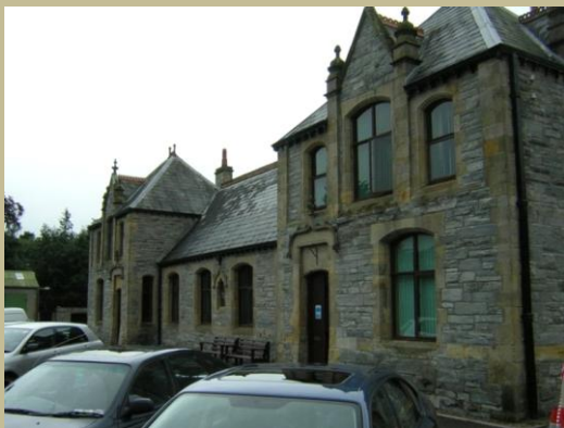
Front Façade of the former Prior School
